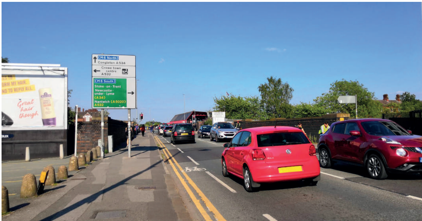
Nantwich Road Bridge
